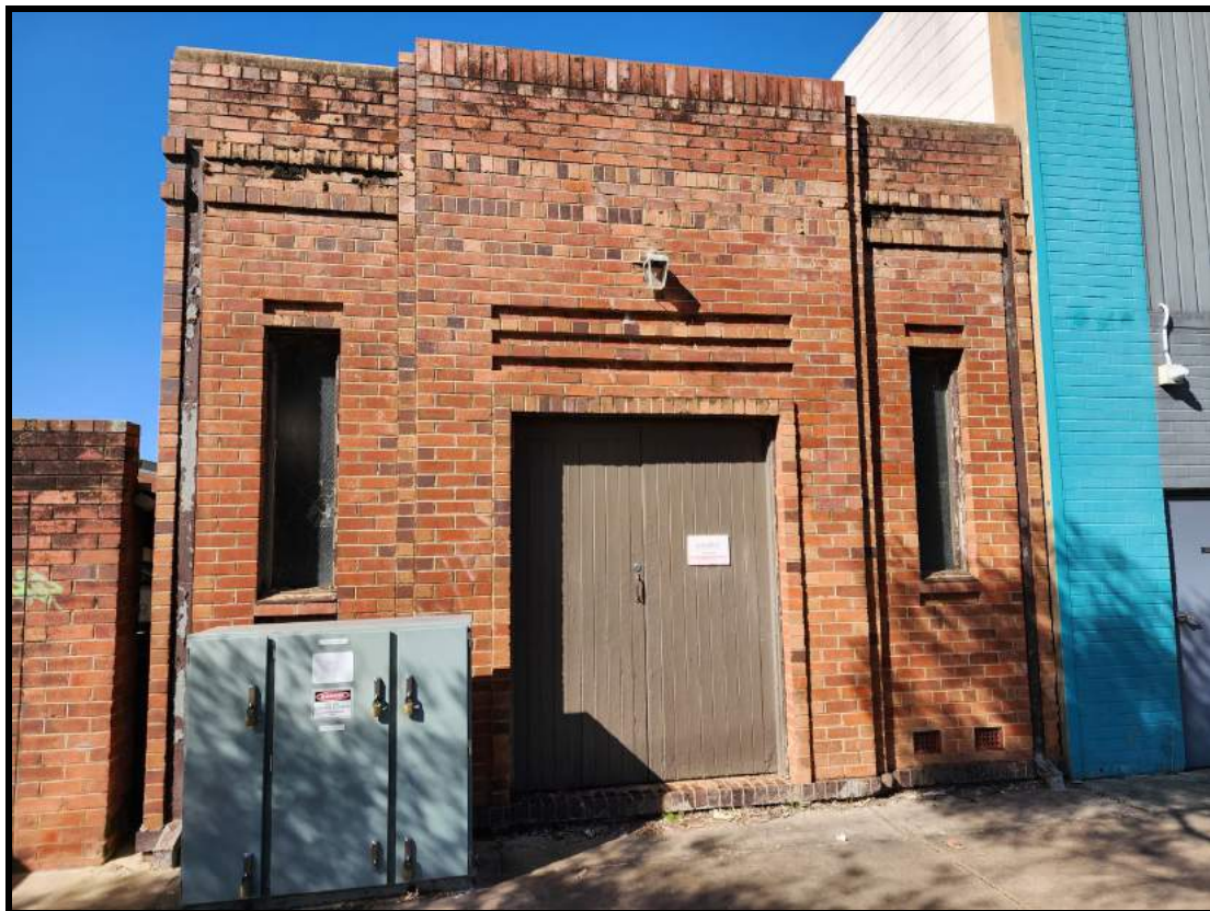
Plate 8: Photograph of electrical substation building.
