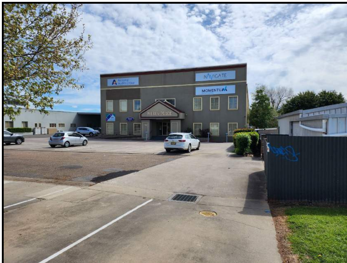
Plate 11: Photograph from Morgan Street toward Piercy Place building.
