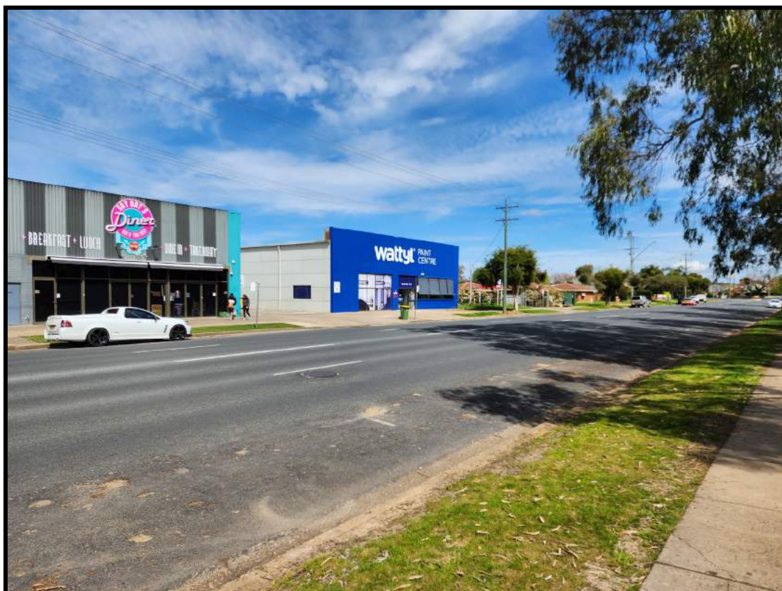
Plate 1: Photograph from Forsyth Street showing front of 2 of large warehouse style buildings.
